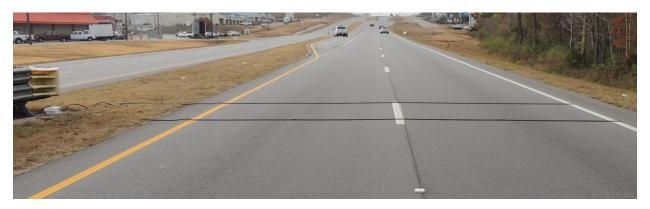
Figure A1. Example of road tubes installation.
