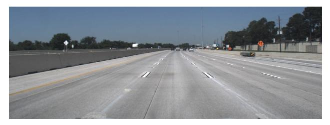
Figure 21: Image of a road segment with white pavement markings with a black border (driving westwards).
