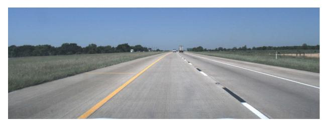
Figure 18: Image of a road segment with white pavement marking followed by black (driving westwards).
