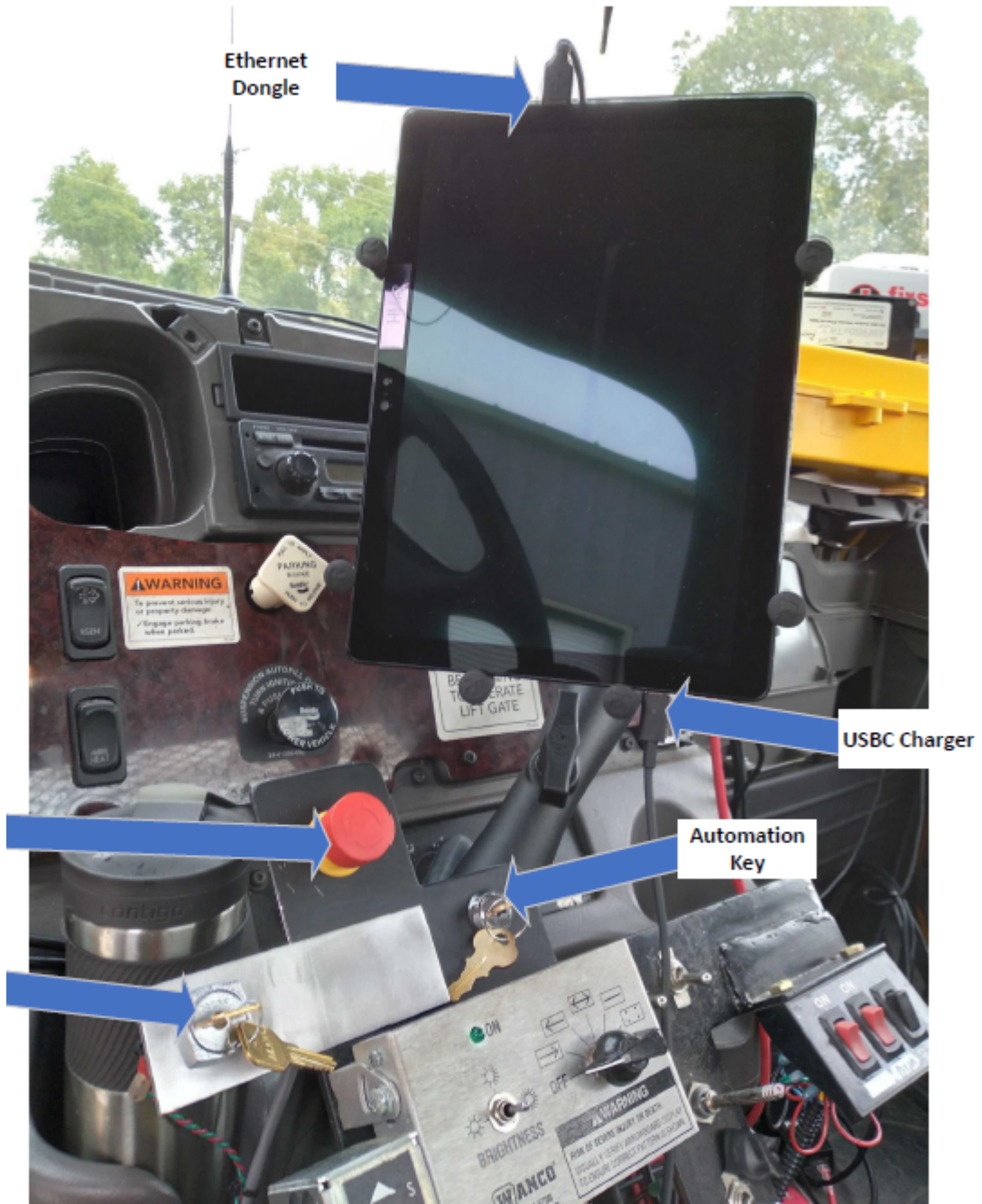
Image 6: Automation keys and Emergency Stop
